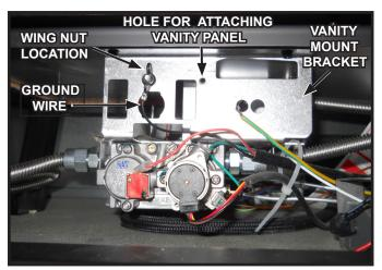
Figure 14.1 Wing Nut on Bracket
