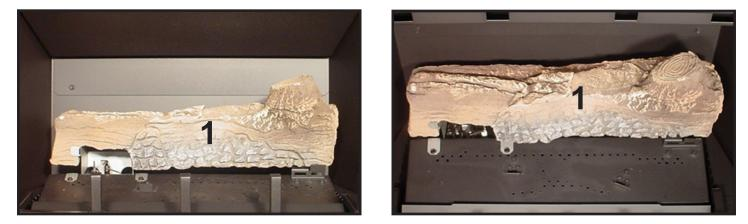
LOG #1 (SRV327-701): Place log #1 at the rear of the unit, with the left edge behind the tab on the pilot bracket. The right side sits behind the tab on the support bracket.
