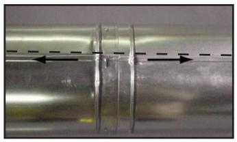
Figure 10.11 Align and Disassemble Vent Sections
