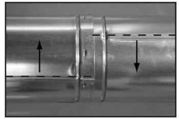
Figure 10.10 Rotate Seams for Disassembly
