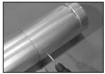
Figure 10.7 Screws into Slip Section
