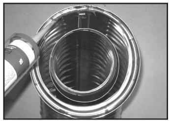
Figure 10.1 High Temperature Silicone Sealant
