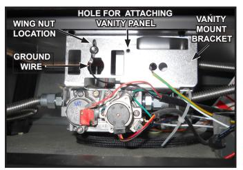
Figure 14.1 Wing Nut on Bracket
