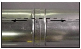
Figure 10.11 Align and Disassemble Vent Sections
