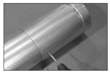
Figure 10.4 - Screws into Slip Section
