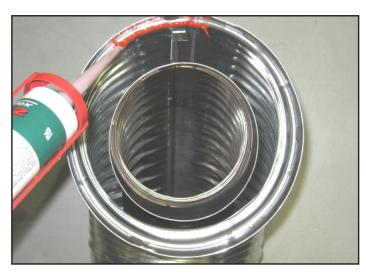
Figure 10.2 - High Temperature Silicone Sealant
