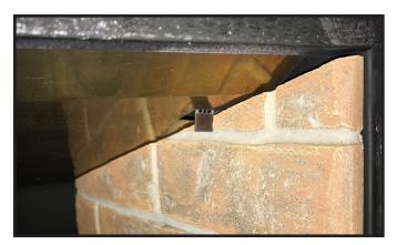
Figure 8. Right Refractory Handbend Tab
