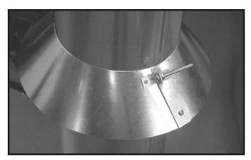
Figure 7.11 insert Bolt into Brackets
