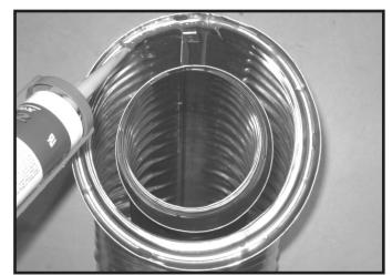
Figure 7.1 High Temperature Silicone Sealant
