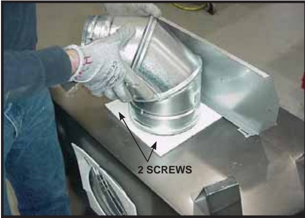
Figure 24. To attach the first section of flue pipe, make sure to use the fiberglass gasket to seal between the first vent component and the outer heater wrap. Use 2 self tapping screws to secure the gasket to the outer wrap.
