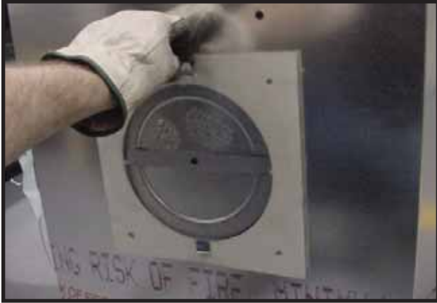
Figure 25. Remove the insulation from the outer flue pipe.
