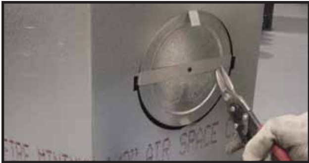
Figure 26. Cut the metal retaining band and fold the sides out.
