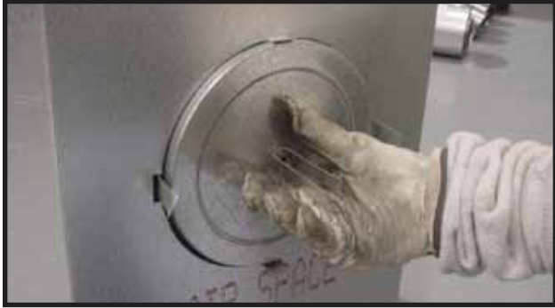
Figure 27. Fold the center parts of the retaining band out and use to remove the flue cap.
