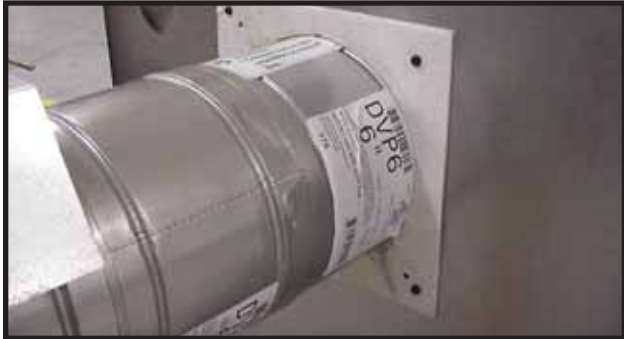
Figure 29. Attach the first flue section (it will snap into place). Slide the insulation gasket onto the flue section, up against the appliance and over the tabs. Use two self-tapping screws to secure gasket to outer wrap.
