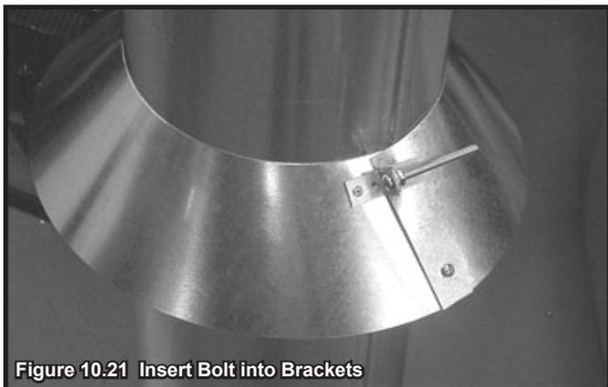
Figure 10.21 Insert Bolt into Brackets
