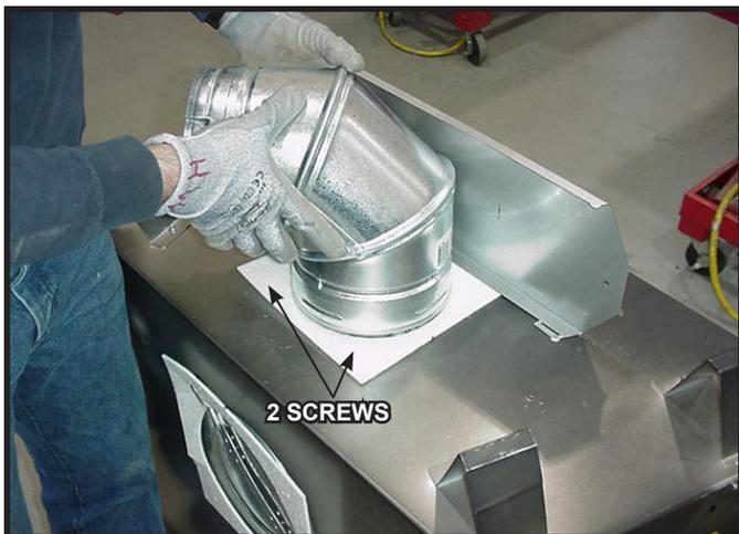
**Figure 9.7** To attach the first section of vent pipe, make sure to use the fiberglass gasket to seal between the first vent component and the outer fireplace wrap. Use 2 self tapping screws to secure the gasket to the outer wrap.
