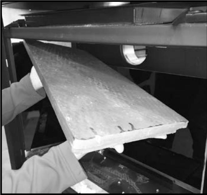
**Figure 11. Install Top Refractory Panel**
