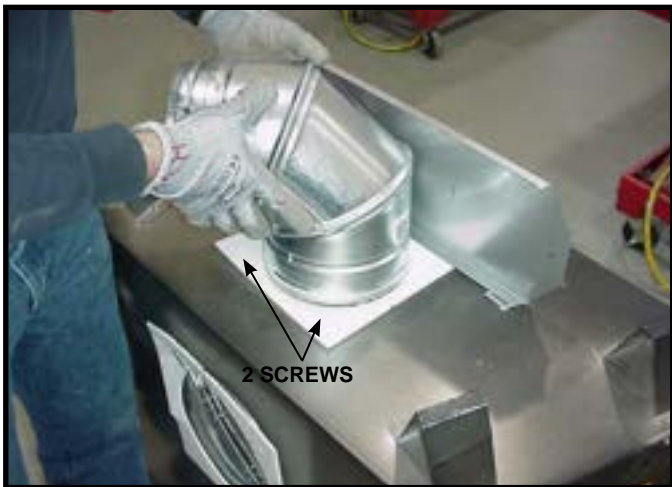
Figure 6.7 To attach the first section of vent pipe, make sure to use the fiberglass gasket to seal between the first vent component and the outer appliance wrap. Use two self tapping screws to secure the gasket to the outer wrap.
