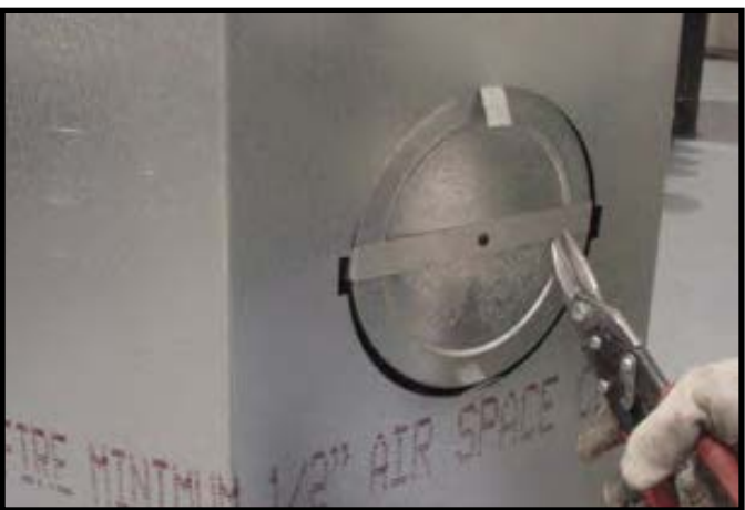
Figure 6.9 (Generic Appliance Shown) Cut the metal retaining band and fold the sides out.
