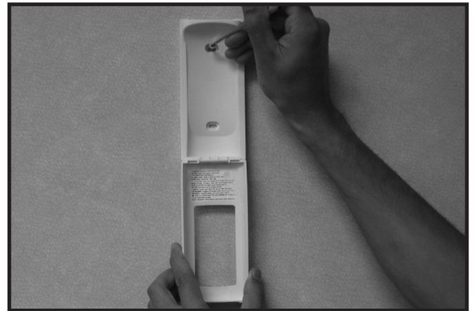
Figure 12.4 Mounting Remote Control Housing
