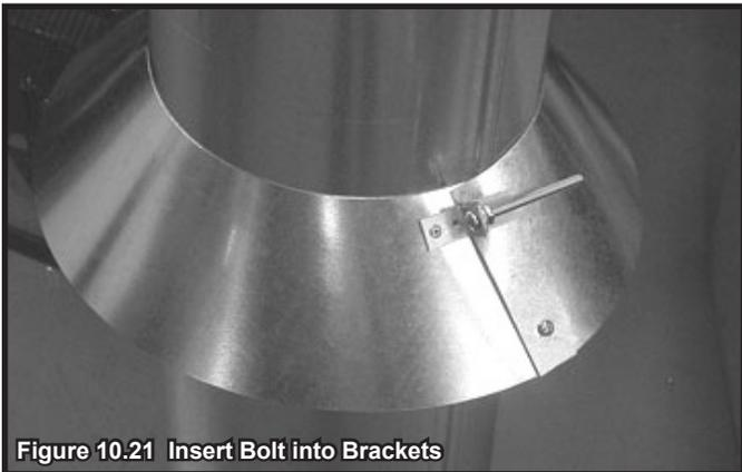
Figure 10.21 Insert Bolt into Brackets
