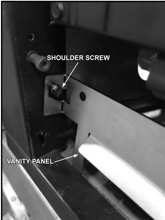
Figure 4 Vanity Panel Installed on Shoulder Screw (Lower Left Corner Shown)
