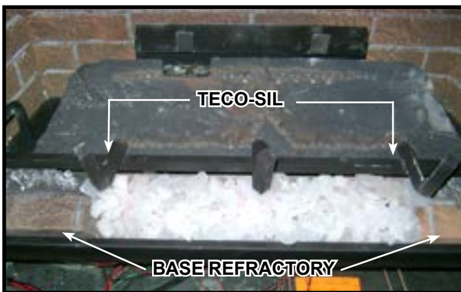
Figure 11.10 Placement of Teco-Sil
