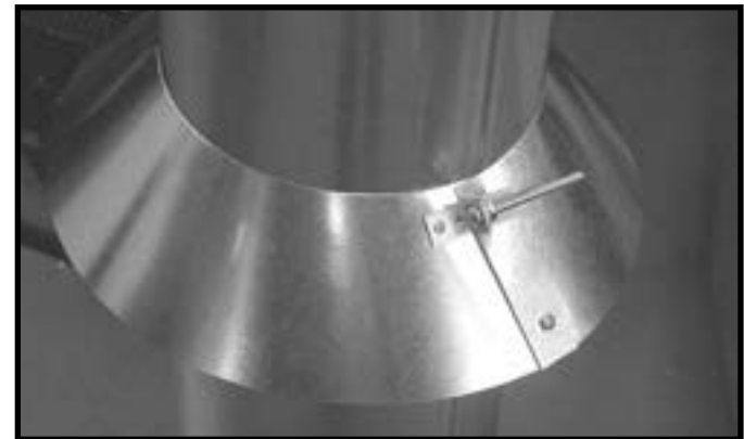
Figure 7.11 insert Bolt into Brackets
