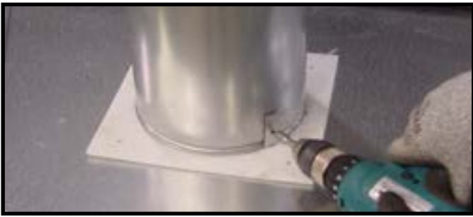
Figure 6.6 (Generic Appliance Shown) To attach the first section of vent pipe, make sure to use the fiberglass gasket in the manual bag to seal between the first vent component and the outer fireplace wrap. Caulk with a minimum of 300 °F continuous exposure rating may be used to hold the part in place.
