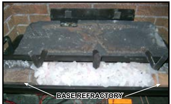
Figure 11.6 Install Base Refractory
