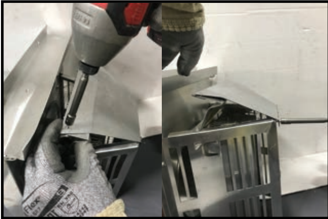
Figure 7.15 Wind Diverter Installed
