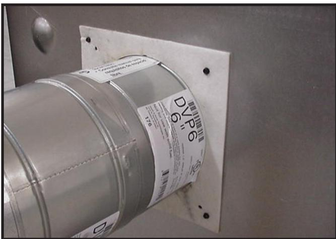
**Figure 6.13** Attach the first vent section (it will snap into place). Slide the insulation gasket, up against the appliance and over the tabs. Use two self-tapping screws to secure gasket to outer wrap.
