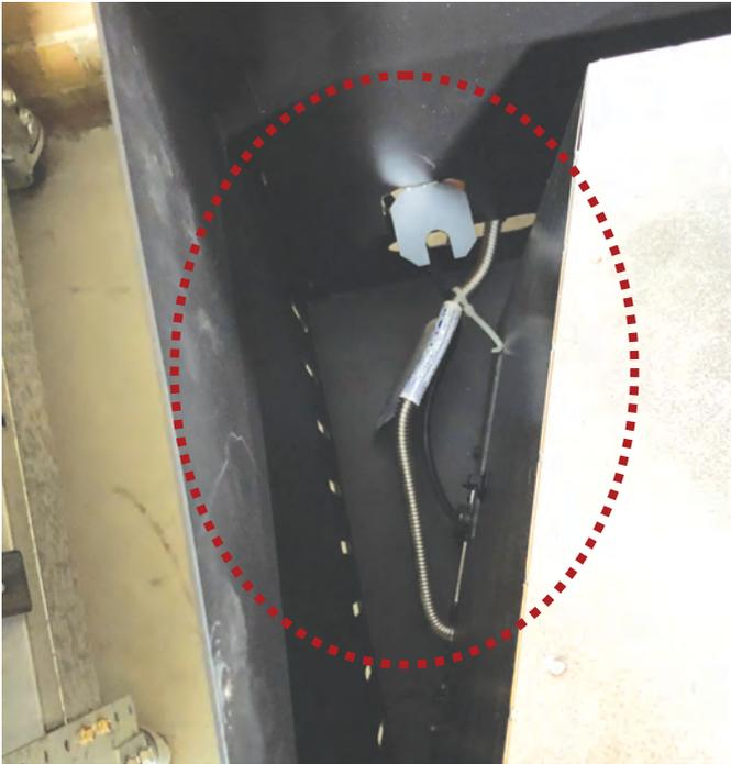
*It is recommended that the bottom 100mm of the i30X unit is sprayed with hi-temp black paint prior to fitting to the freestanding case. This is to ensure no silver metal is visible through the ventilation slots on the side of the free standing casing.*
