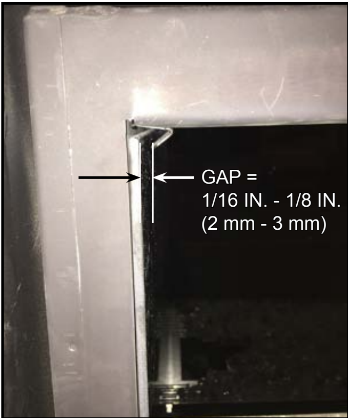
Figure 11.9 Gap Between Tab and Side Glass Panel: 1/16 IN. - 1/8 in.
