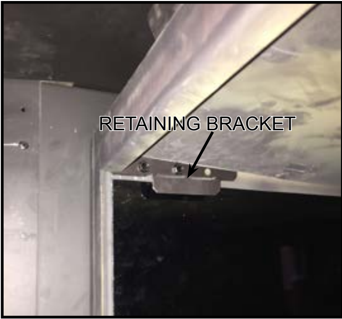
Figure 11.8 Retaining Bracket Installation - Side Panel
