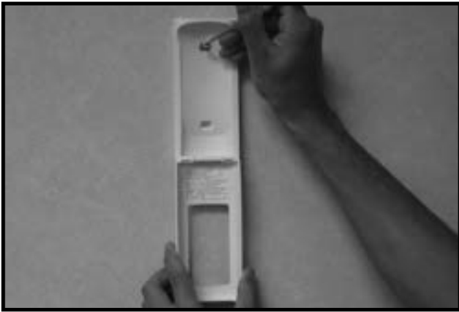
Figure 3.8 Mounting Remote Control Housing
