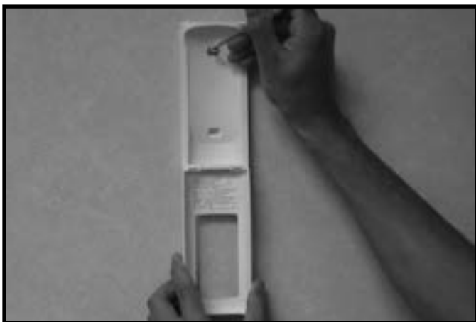
Figure 3.8 Mounting Remote Control Housing
