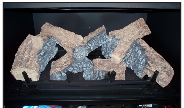
Figure 9. Log Set Installed
