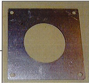
Flue baffle restrictor plate fitted to flue outlet
