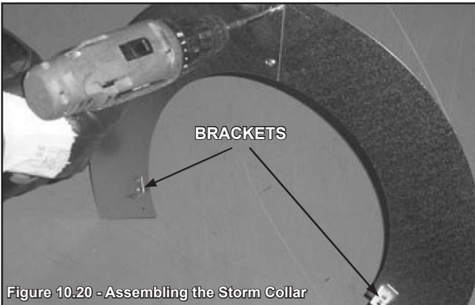
Figure 10.20 - Assembling the Storm Collar
