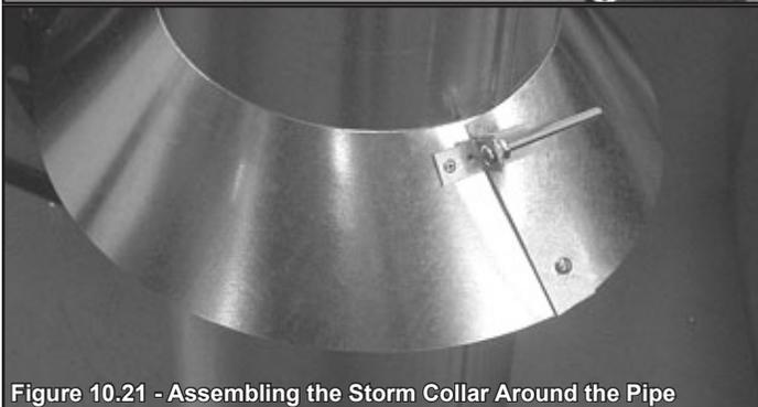
Figure 10.21 - Assembling the Storm Collar Around the Pipe
