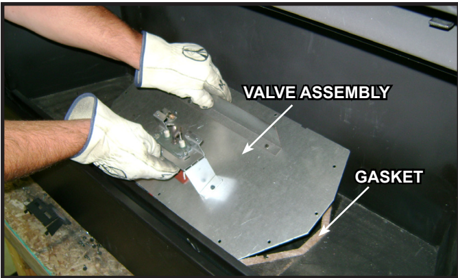
Figure 16.6 Remove Valve Plate
