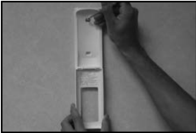
Figure 3.11 Mounting Remote Control Housing
