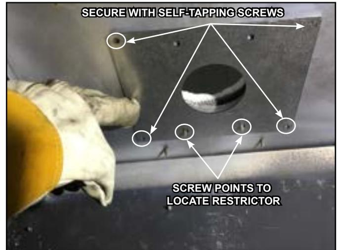
Figure 5.9 Natural Gas Restrictor Plate
