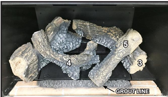
Figure 16. Log #5 Installed
