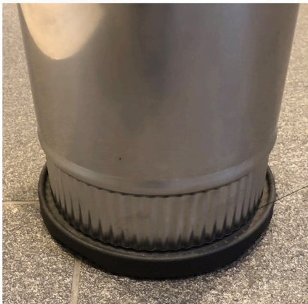
Flue seated correctly.
