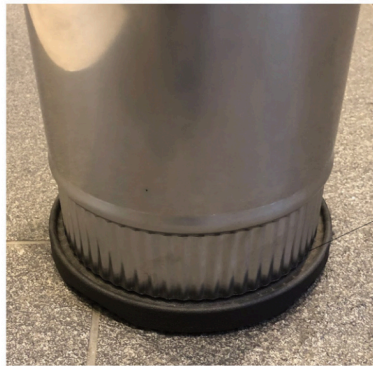
Flue seated correctly.
