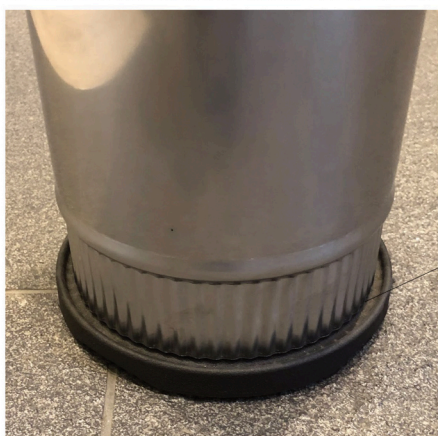
Flue seated correctly.
